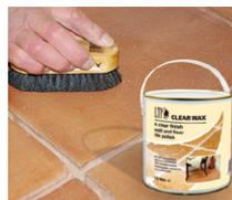
Leave to dry for 24 hours. Apply a light coat of LTP Clear or Antique Wax using a soft cloth. Buff with a soft brush.
