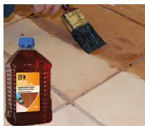
Saturate with LTP Boiled Linseed Oil. Remove any excess that remains on the surface an hour after each application.
